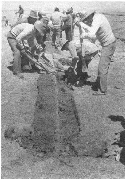
6 (above) Members of the Community of Segunda Collana using footplows to cut sod blocks from old canals for the retaining walls for rebuilding the raised field platforms in Viscachani Pampa, Huatta (October 1985).
